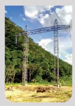
GANTRY TOWER ERECTED ALONG 220KV KIDATU-IRINGA LINE AT IYOVI.
