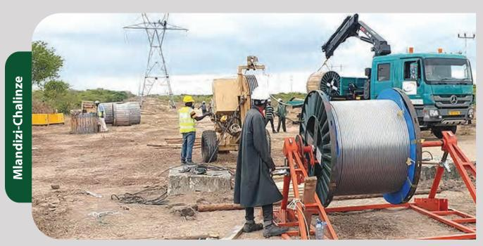
$\label{prop:conductors} \textit{Preperation and rolling of conductors during the replacement of old ones.}$
